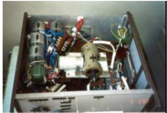
Fig. 3. Power pack and control system for high voltage discharge system.
