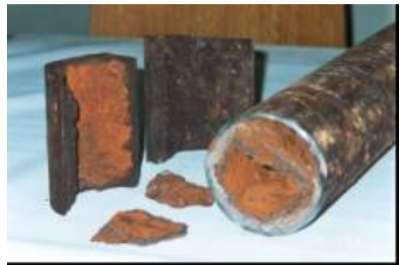
Fig. 17. View to tube from full rust
